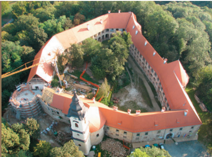
The view on the castle and the castle's courtyard during the renovation and archaeological excavations in the year 2004.
